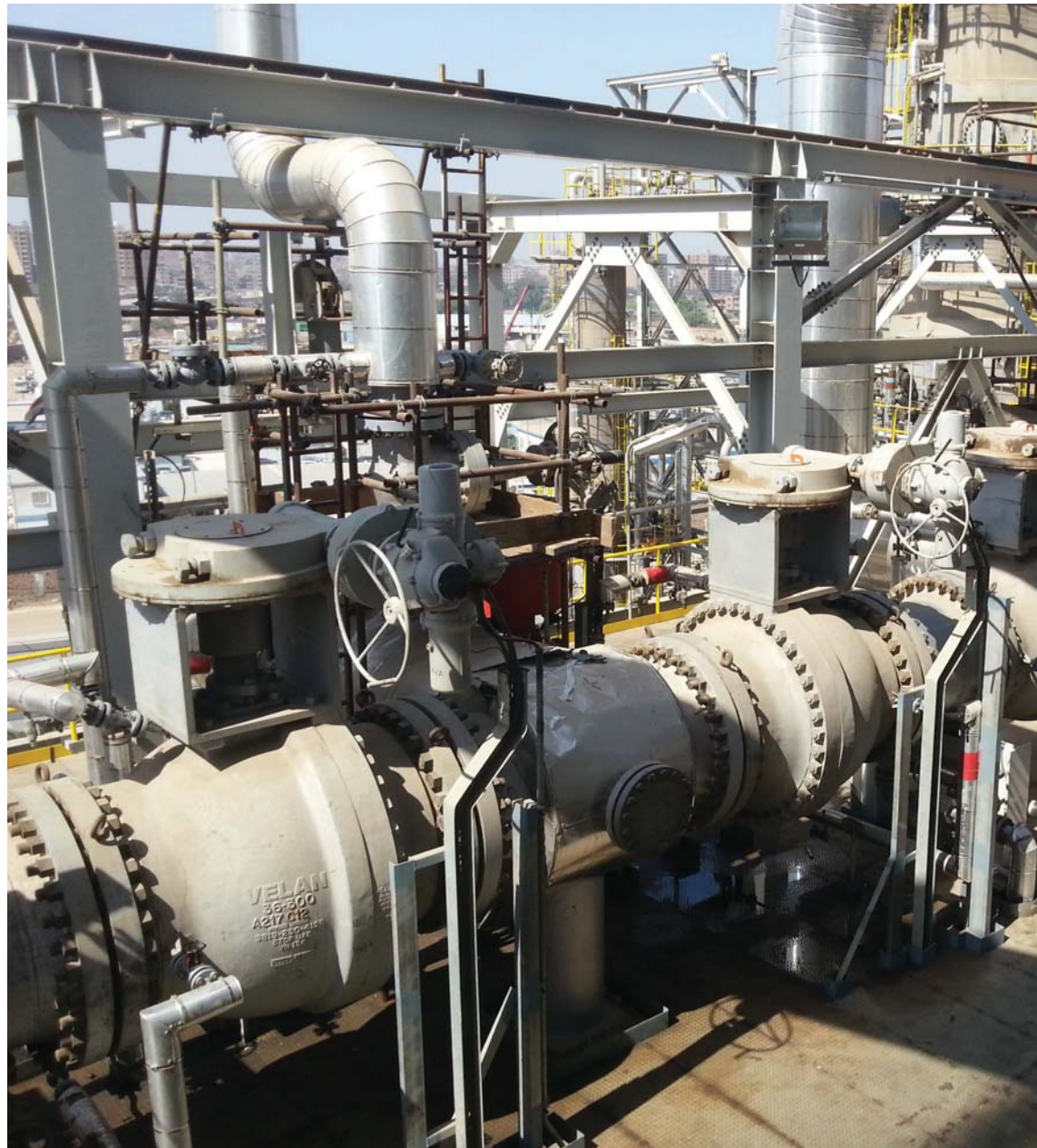
Three 36" Class 300 two-way severe service metal-seated ball valves installed at a refinery in Egypt.
