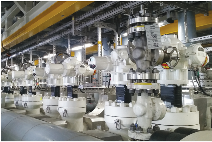
Rotork intelligent actuators have been installed on the all-electric Johan Sverdrup platform
