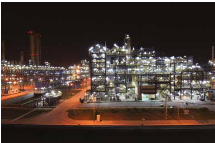
Dow's production facility in Zhangjiagang.
