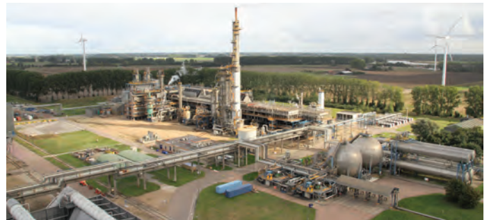
Zooming in on the ammonia plant.
