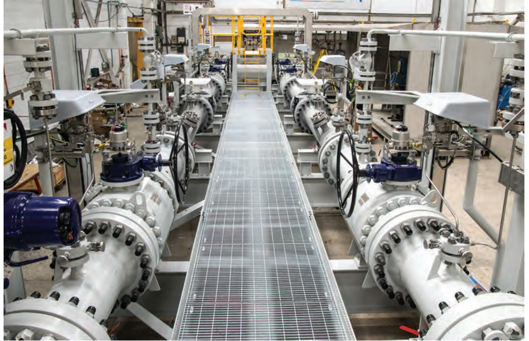
Metering system with condition based monitoring. These systems are designed to monitor critical equipment to avoid unexpected outages and downtime.
