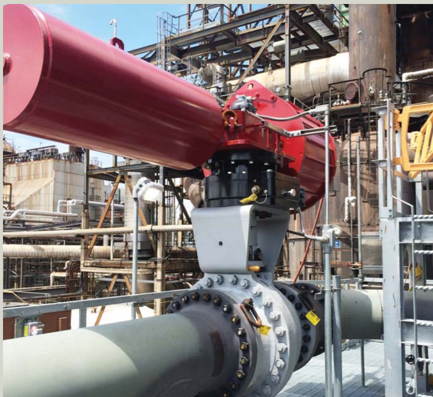
20" (500 mm) Class 300 Securaseal R-series cast valve in service
