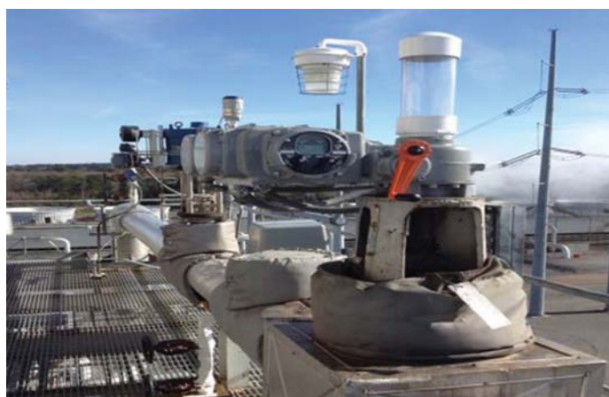
Hard to reach and remote locations are typical for Emerson's EIM electric actuators.
