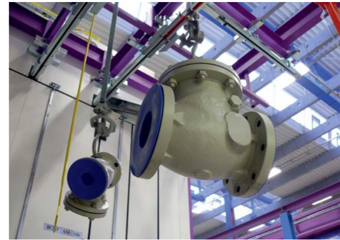
Swing check valves being coated.
