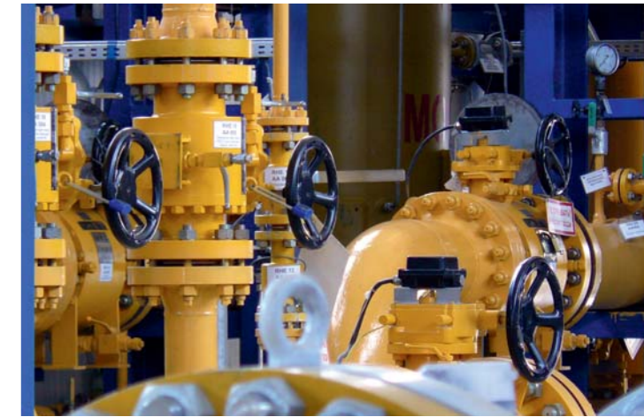
Power plant installation in Kaliningrad.
