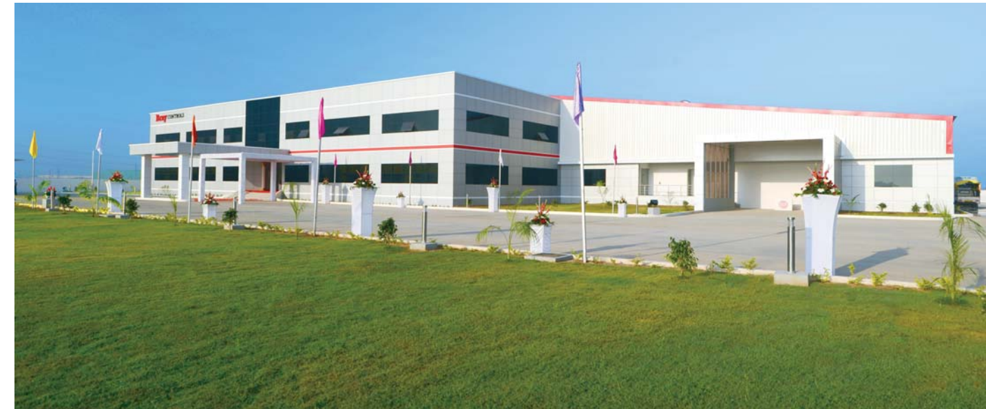
Bray International Manufacturing Facility – Vadodara, India
