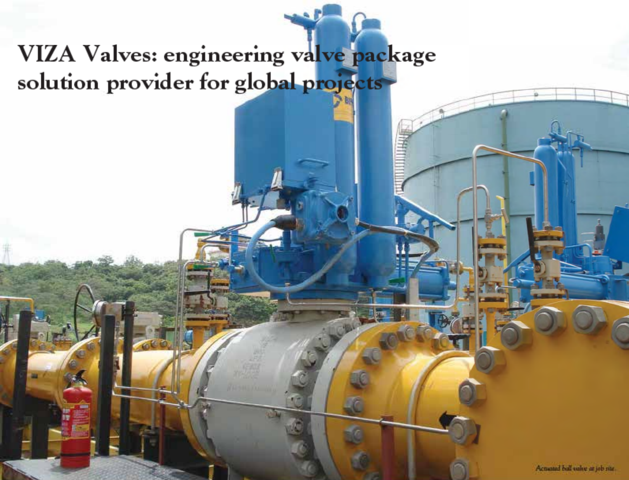
Motor actuated metal seated ball valve
