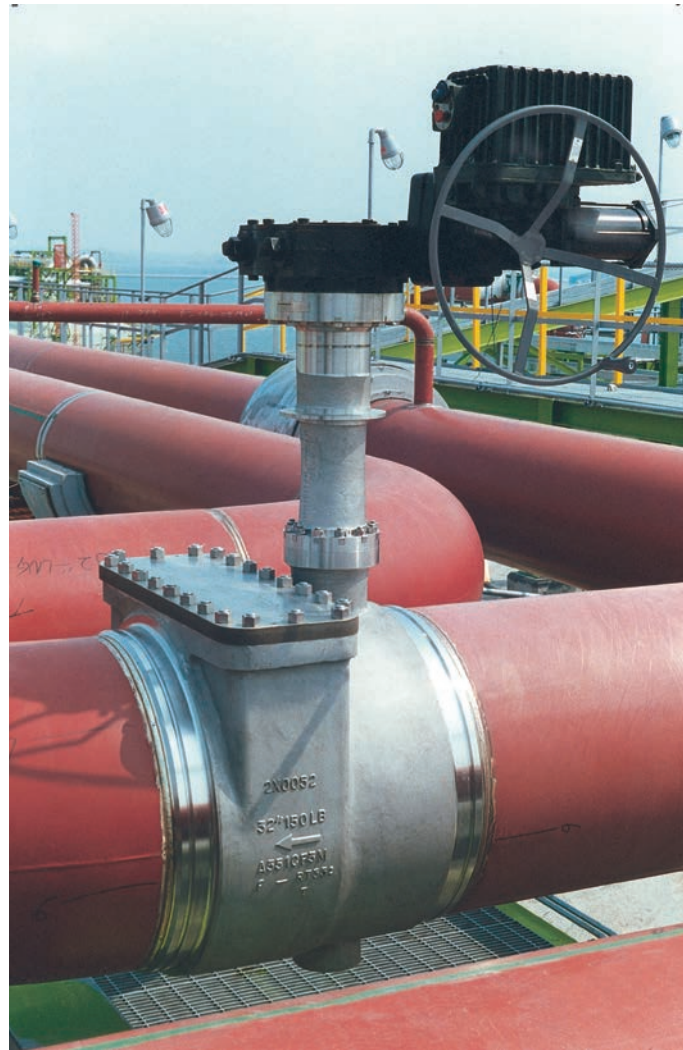
Velan Velflex High Performance Butterfly Valves have been used in LNG receiving terminals for over 20 years.
