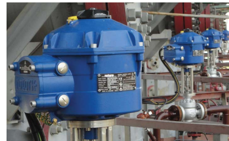
CVA electric control valve actuators recently installed at a Ukrainian compressor station on the pipeline network supplying Western Europe with natural gas from Russia and Central Asia.
