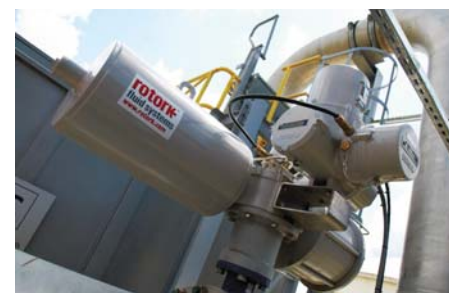
Rotork Skilmatic electro-hydraulic failsafe actuator installed for safety-related valve duty at the Vopak Europoort Terminal in Rotterdam.
