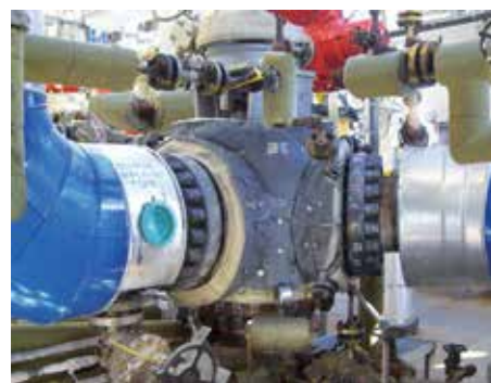
A Velan coker switch valve in service in a European refinery. Velan is a leading supplier of coker ball valves worldwide.
