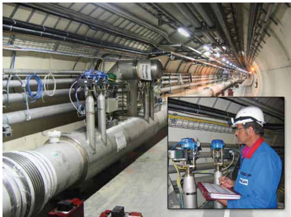
The Large Hadron Collider (LHC) at CERN (European Council for Nuclear Research), Geneva. The LHC is the world's largest, fastest, and coldest accelerator of nuclear particles. Currently, it has over 2,500 Velan bellows seal cryogenic valves installed and controlling the flow of over 700,000 litres of liquid helium.
