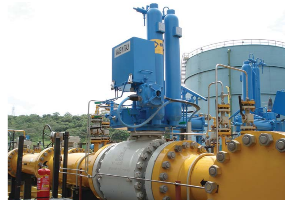
Actuated ball valve at job site.
