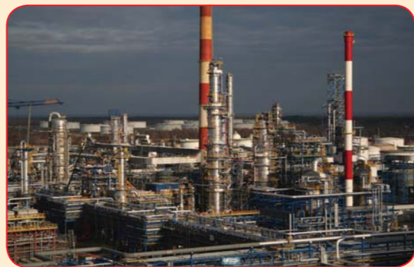
Aerial shot from the Grupa LOTOS refinery.
