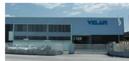
Velan ABV S.p.A., Head Office and Plant 1 Lucca, Italy.
