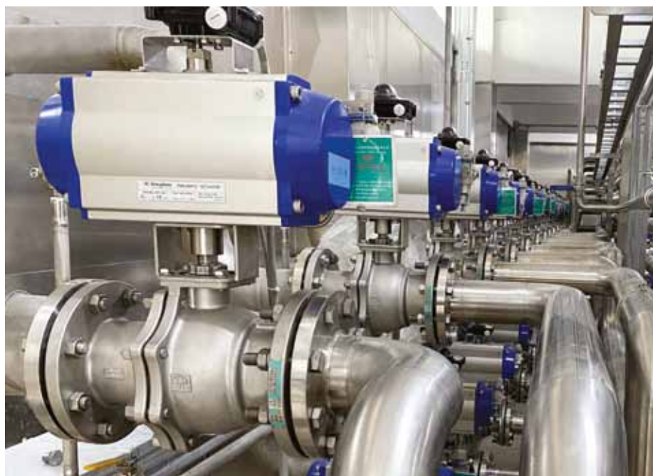
Automation application with KI ball valves and KI pneumatic actuator.
