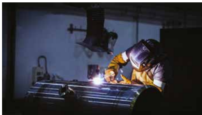
Welding in progress of desuperheater
